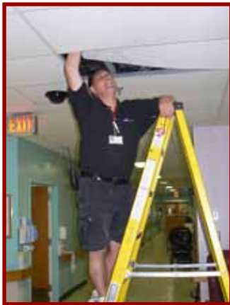
Ernie Montour making repairs in Inpatient Department
